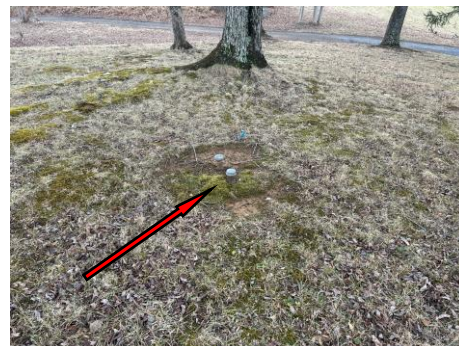
Buried oil tank right side of house.
