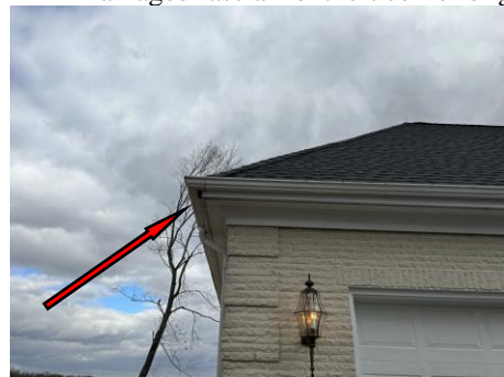
Recommend chimney flue caps. Damaged fascia front left corner of garage.
